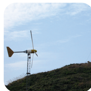
Windpower installation in China Source : Bergey Windpower
